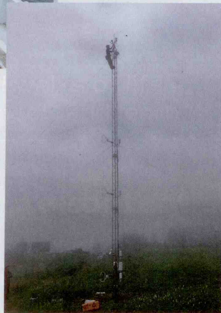
Alexi Perelet, a trained graduate student from the University of Utah, climbs the 15-m flux tower for C-FOG to mount an infrared gas analyzer and sonic anemometer. (PHOTO: Sebastian Hoch)
